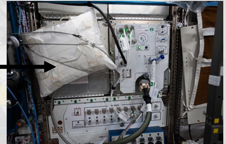
SERFE Flight Unit installed on ISS. 1
