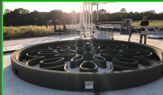
Terrestrial printing of cementitious material
