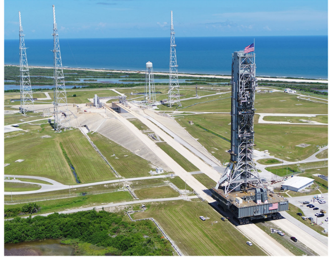
b) Aerial view of Mobile Launcher
