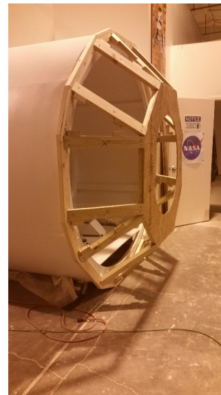
Fabricated end cap and installed window
