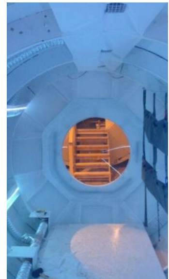
Installed interior and aesthetic components
