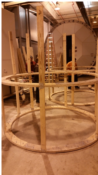
Attached and assembled structural shell
