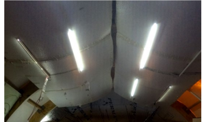
Former Lighting in MPLM
