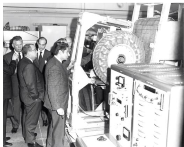
Figure 4: NASA Low Gravity LRV Test Apparatus Interior and Exterior
