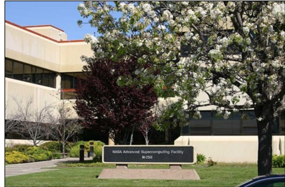
NASA Advanced Supercomputing facility at Ames Research Center.
