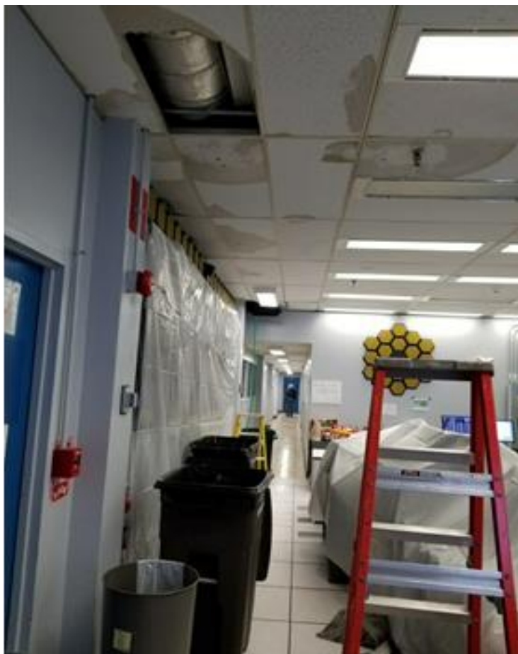
Water Damage in B32 OTIS Control Room, despite pre-test roof repairs
