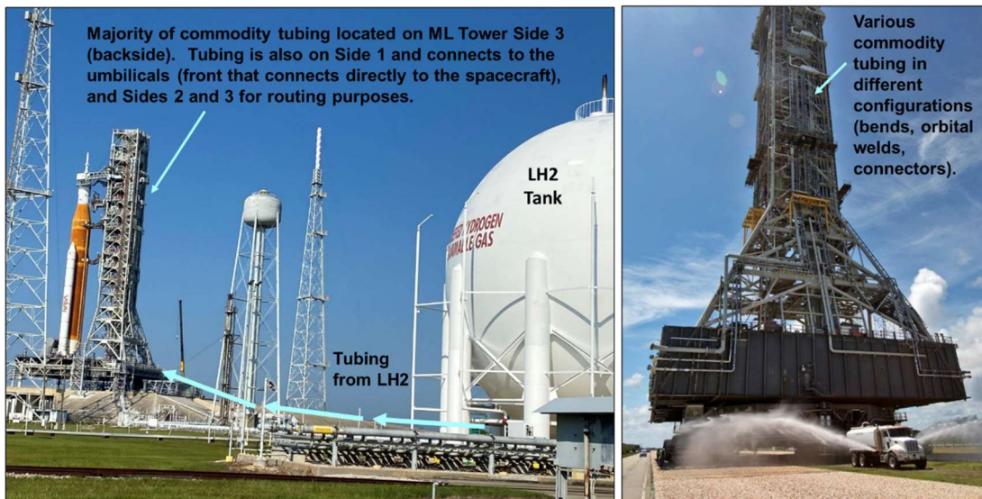
Figure 2: Examples of commodity tubing at Launch Complex-39B with Mobile Launcher 1.
