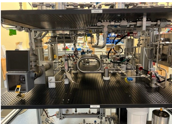
Middle Deck of RFC Breadboard Fuel Cell Cart
