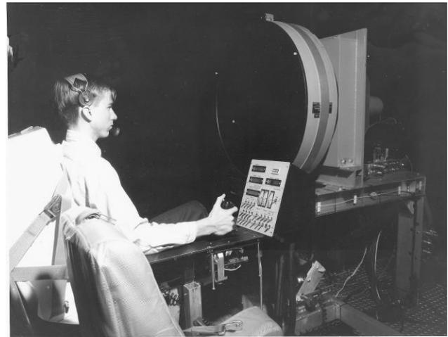
Figure 3. A subject using an Apollo type vertical pistol grip controller in an LRV simulator with a large circular TV monitor display [5].
