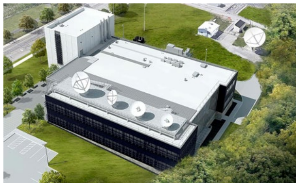
Fig. 1. The Aerospace Communications Facility at NASA Glenn Research Center, which opened in August 2023
