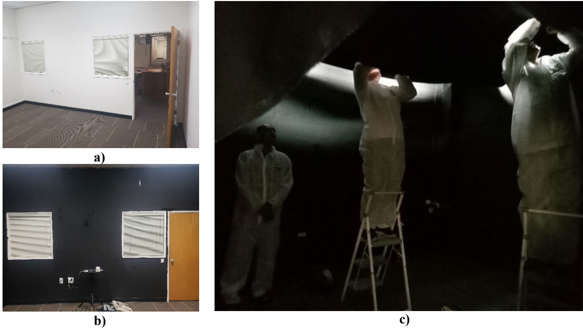
Fig. 9 LAE Environment darkroom outfitting: a) LAE prior to flat black paint application, b) flat black paint applied to walls of LAE, and c) black vinyl fabric attached to ceiling to inhibit diffuse lighting.
