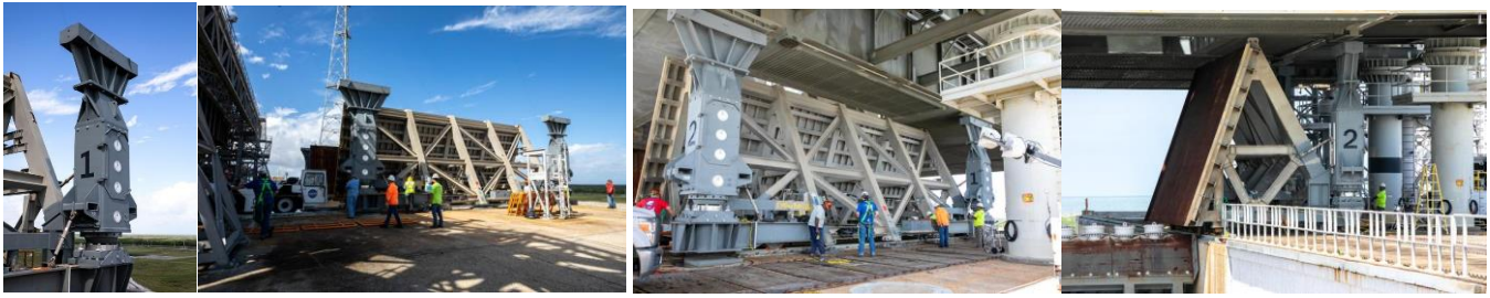
Figure 2. Launch Pad 39B extensible columns and side flame deflectors
