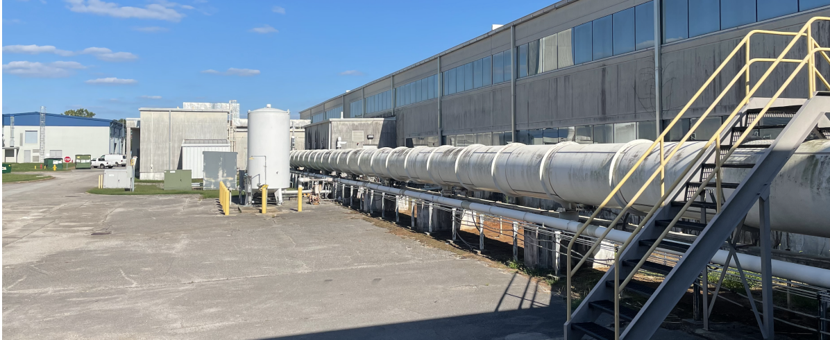
Figure 1. The Marshall 100-Meter X-ray Beamline, located at Marshall Space Flight Center adjacent to Building 4487 and has a total line length of 101 m. Also known as The Stray Light Test Facility, this installation was constructed in 1963 and is used extensively both for MSFC internal optics development and the broader scientific community as made available through APRA.
