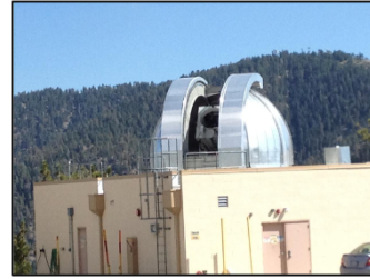
OCTL Ground Station
