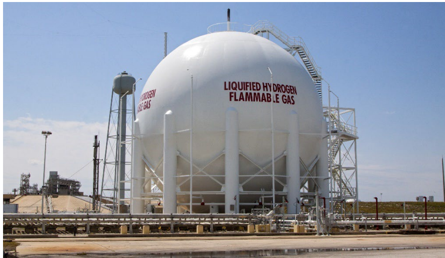
Figure 1.1 Liquid hydrogen tank (LH2) tank at LC-39B at KSC
