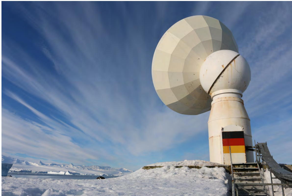
Fig. 1 View of the 9-meter radio telescope at GARS.
