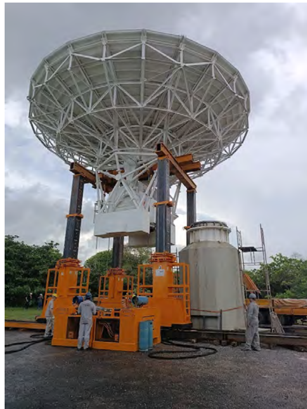
Fig. 2 The 14.2-m antenna set down off the pedestal for bearing replacement activity.
