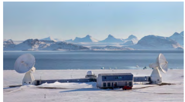
Fig. 2 The geodetic observatory's Brandal site with 13-m twin telescopes. From left to right: Ny-Ålesund 13-m North antenna (Nn), SLR dome, operations building, and Ny-Ålesund 13-m South antenna (Ns). (Image: Bjorn-Owe Holmberg)
