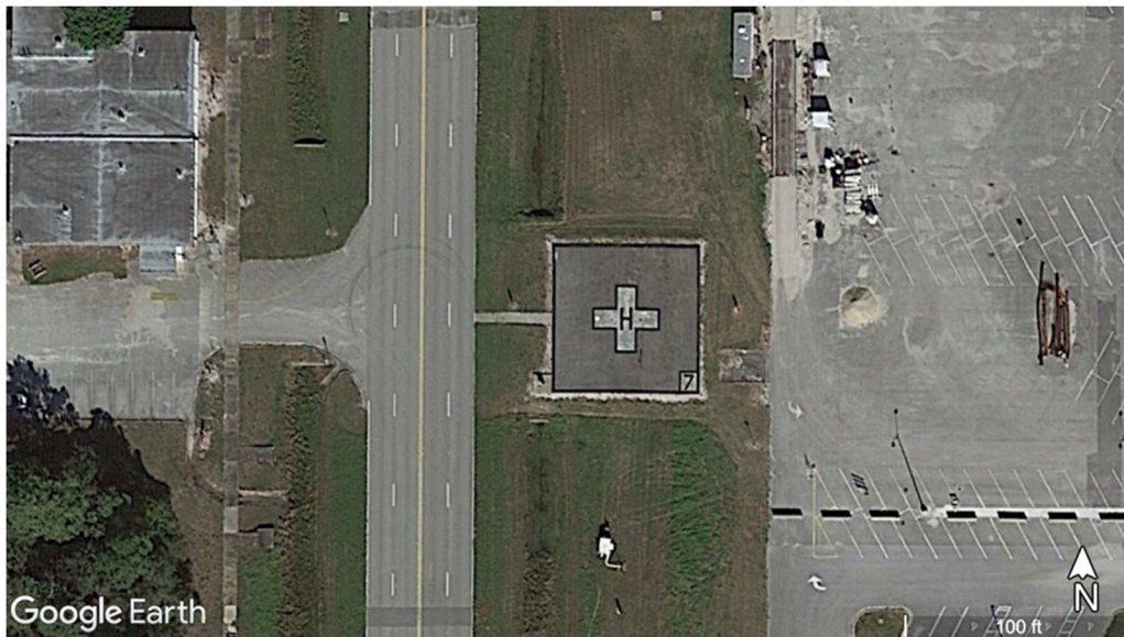
Fig. 7 Google Earth overhead view of the Operational Health Facility helipad at the Kennedy Space Center.
