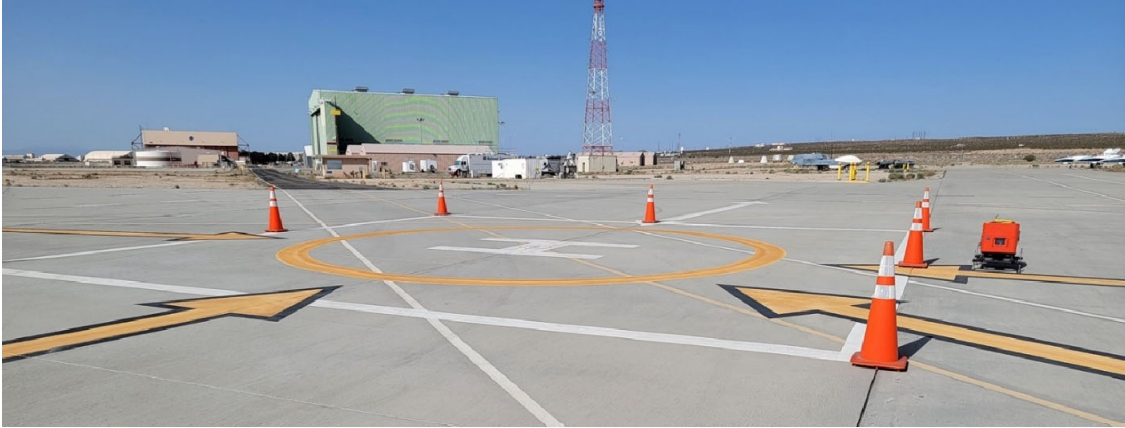
Fig. 8 Photograph taken facing southwest of the TLOF marked with traffic cones and adjacent PLASI (right). (Photograph courtesy Nelson Brown, AFRC.)
