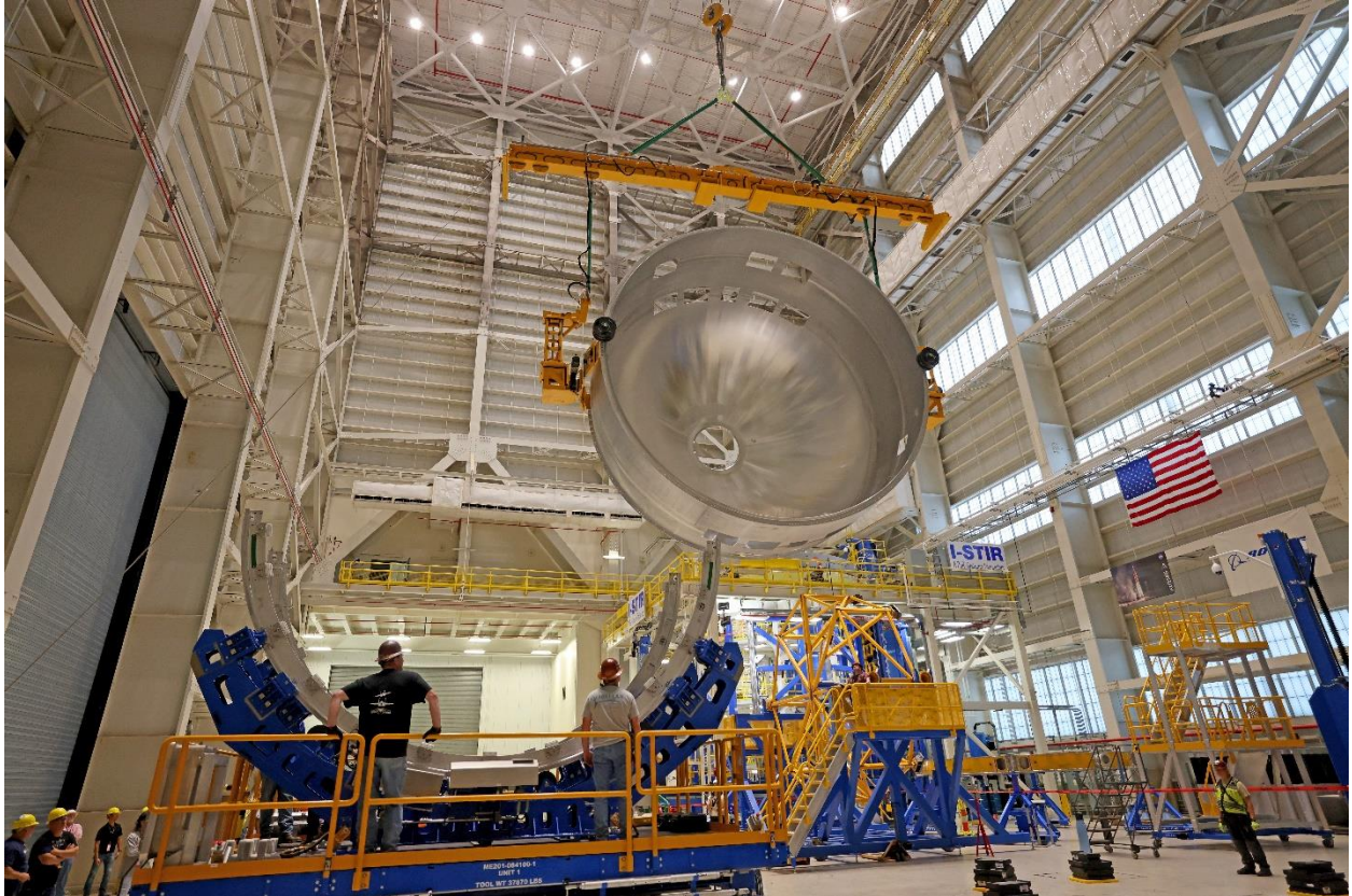
Fig. 7 A LOX dome for the EUS weld confidence article, above, was manufactured at Michoud. The WCA is being built now.
