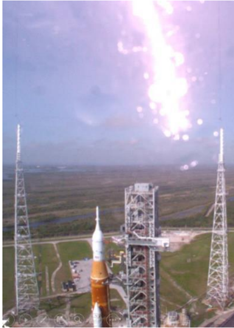
Figure 10: Lightning striking the Lightning Protection System on April 2, 2022. [Photo: NASA]
