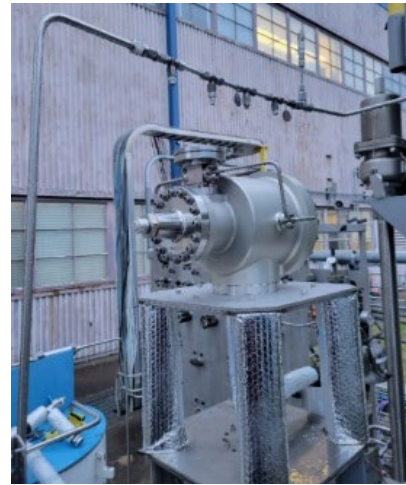
Fig. 13: CDA Spraybar Setup
