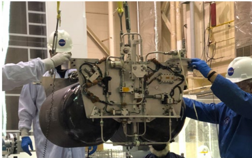
Fig. 4 LOFTID's Updated Pneumatics Plate
