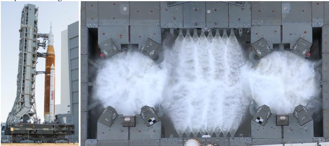
Fig. 1 SLS vehicle on the mobile launcher (left) and the mobile launcher IOP/SS water system (right).
