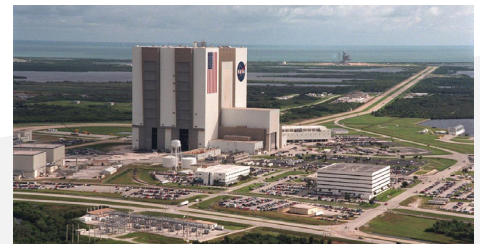
Figure 33: The Kennedy Space Center in Merritt Island, Florida.
