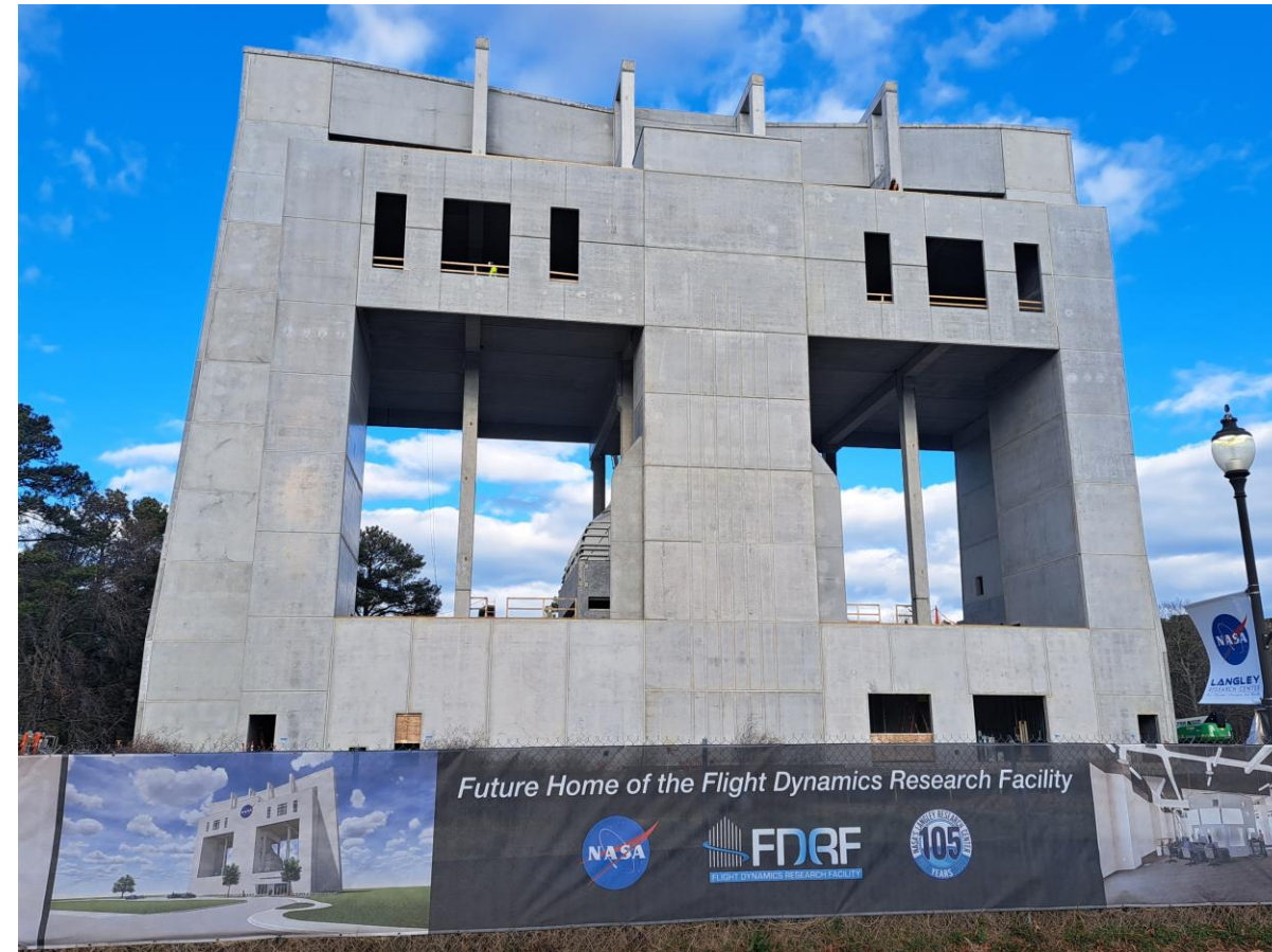
FDRF construction progress (Dec. 19, 2023)
