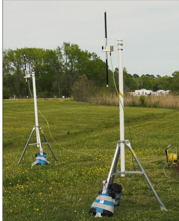
Figure 29: uAvionix microLink Receiver on CERTAIN (Temporary Installation)
