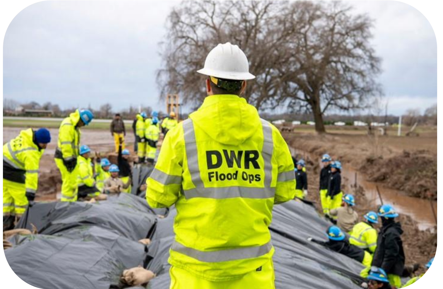
Image Credit: Kenneth James, repair work of levee breach on Deer Creek
