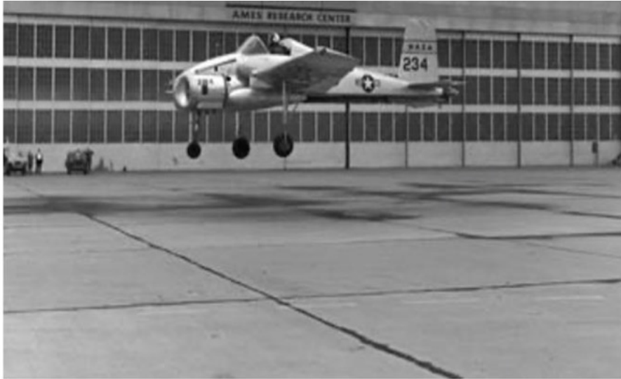
Bell XV-3 (experimental tilt rotor)
