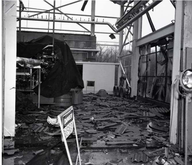
Damage at Lewis' Rocket Engine Test Facility following a test of high-energy fuels (4/27/1955)
