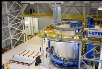
LH2 tank in progress
