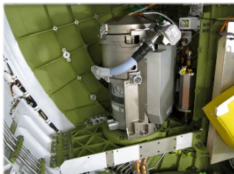
Figure 1. Orion UWMS installed in Artemis-II Vehicle
