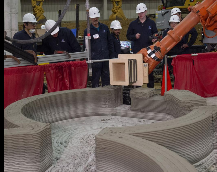
Penn State 3D prints a cementitious habitat prototype
