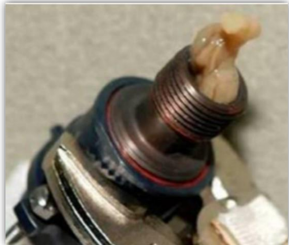
Figure 2: Biofilm accumulation in piping 2
