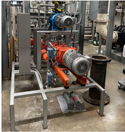
Figure 5. New 20 FT Busch Vacuum Pumps
