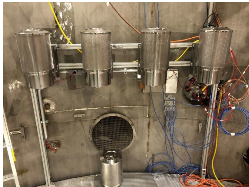
Figure 7. 20 FT Air Revitalization System, 1 st Floor
