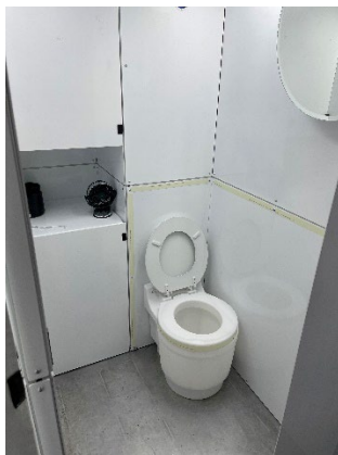
Figure 8. 20 FT 2 nd Floor Laveo® Dry Flush Toilet
