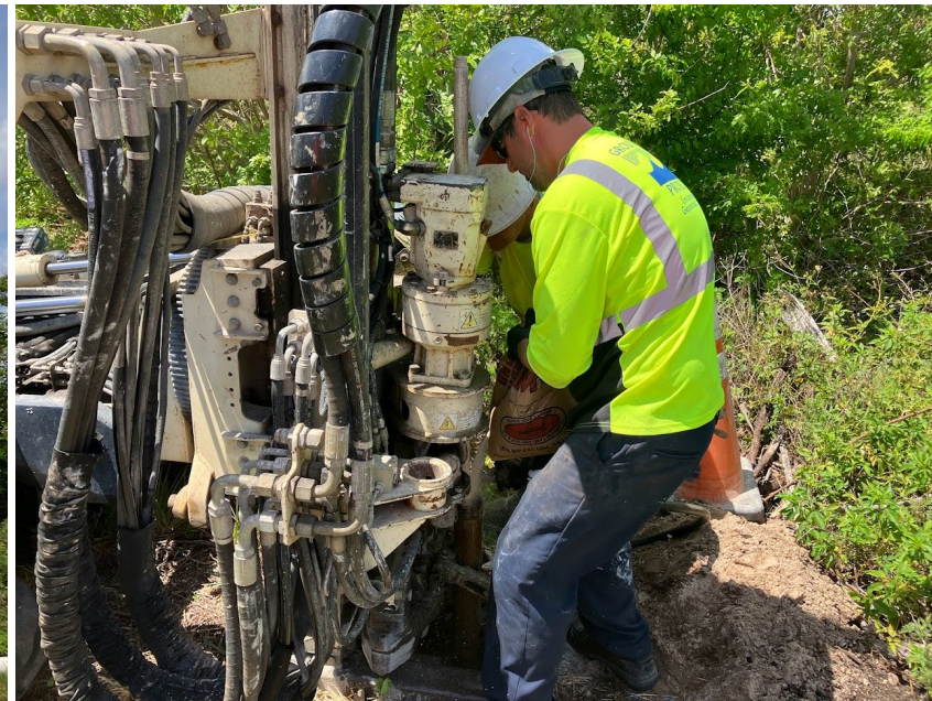
Photo of driller adding 20/30 silica sand for filter pack.
