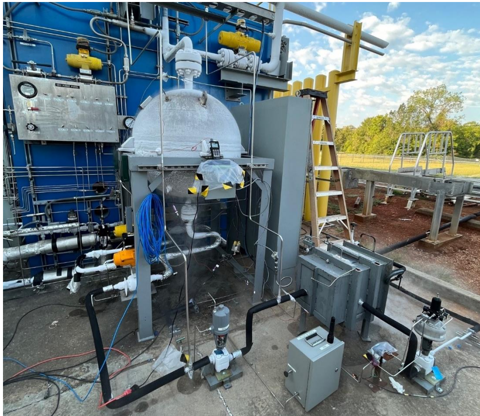
Figure 3. Cryogenic pressure cycle test setup
