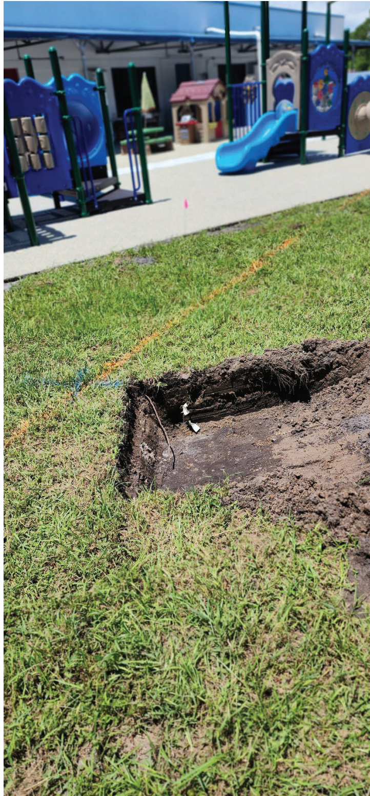
Figure 2: Photo of Excavation to be Sampled: August 3, 2023
