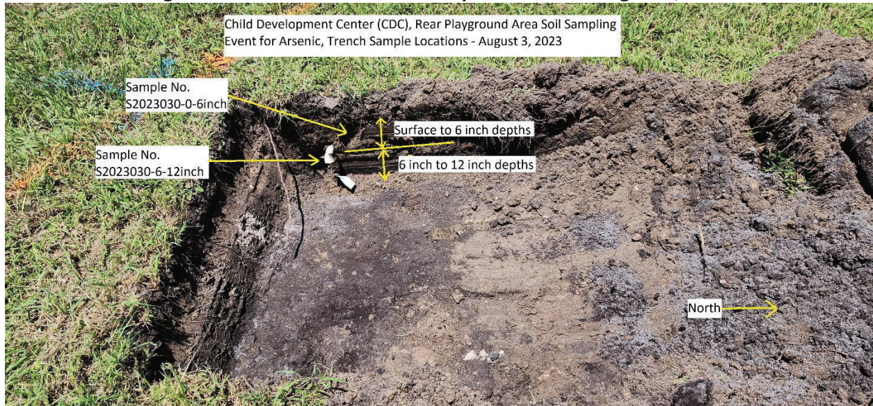
Figure 4: Photo of Excavation Sample Locations: August 3, 2023
