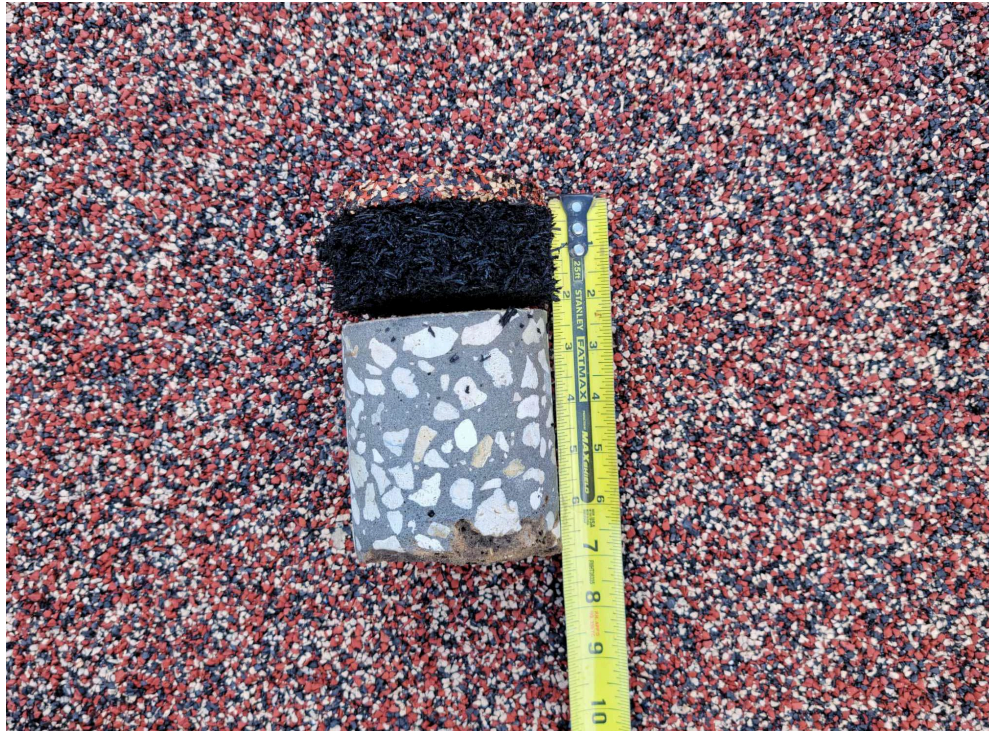
Playground surface and concrete core from KCDC-SB0046.
