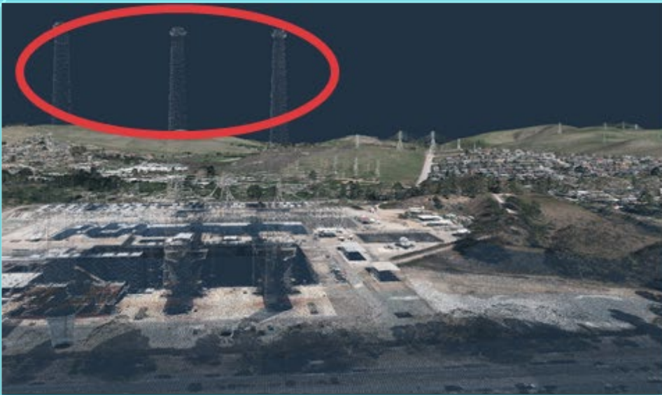
Holes and Gaps
