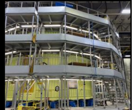
Intertank in progress
