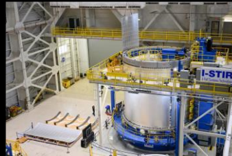
LH2 tank in progress
