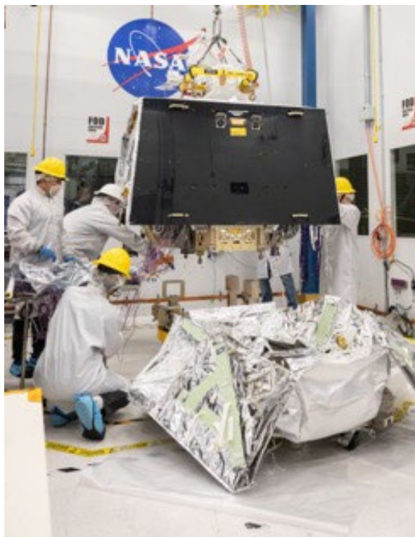
Fig. 8: VIPER solar arrays being installed.
