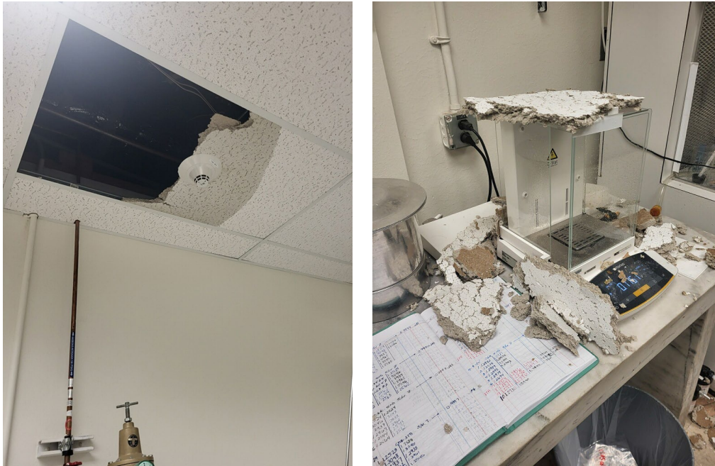
Figure 6. Ceiling Tile Collapse Causing Temporary Disruption in Workflow Note the flow bench to the right of the balance.
