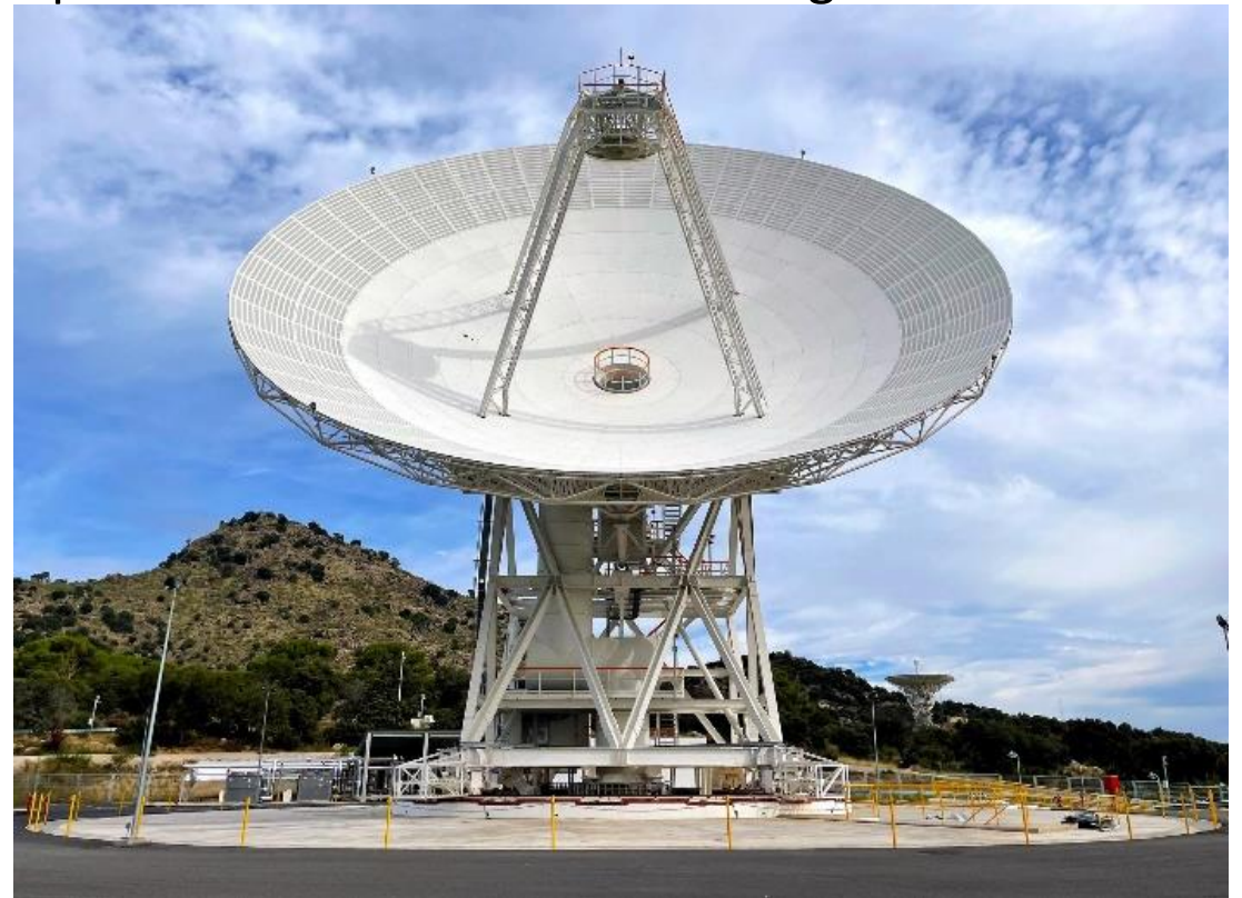
Deep Space Station 53 is a new waveguide antenna that went online in February 2022 at NASA's Deep Space Network's ground station in Madrid.
