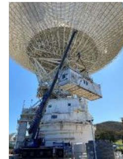
Pump House removal
