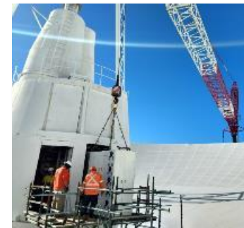
S400 klystron cabinet removal
