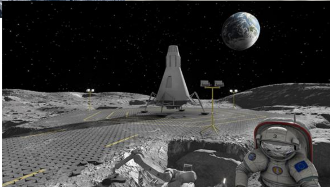
Vision of ESA's PAVER Concept of a Paved Road and Landing Pad Area Using Interlocking Triangular Pavers. Image from ESA
