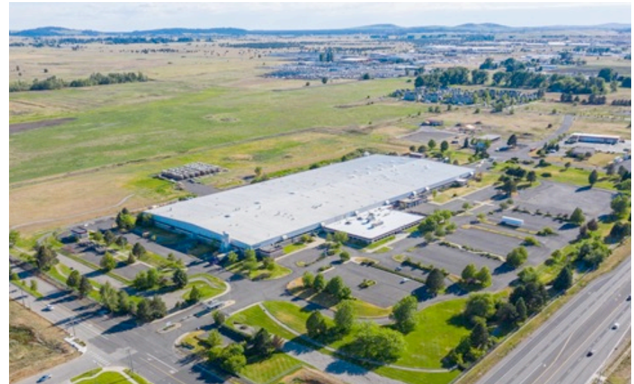
In Spokane WA at vacated Triumph facility
