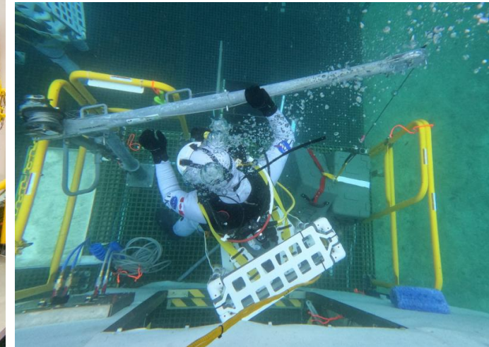
Davit boom causing porch maneuverability issues.
