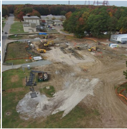
(b) Foundation construction, Nov. 2022
