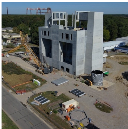
(g) Before test section install, Oct. 2023
