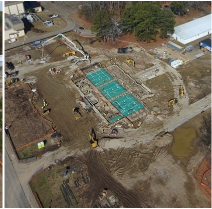
(c) Slab placement, Feb. 2023
