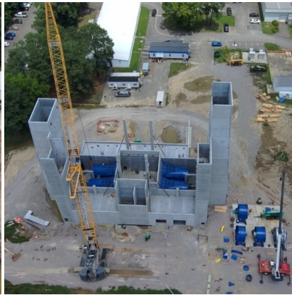
(e) Fan installation, July 2023
