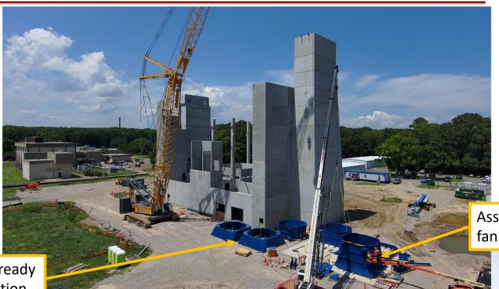
Assembly of fan diffusers
